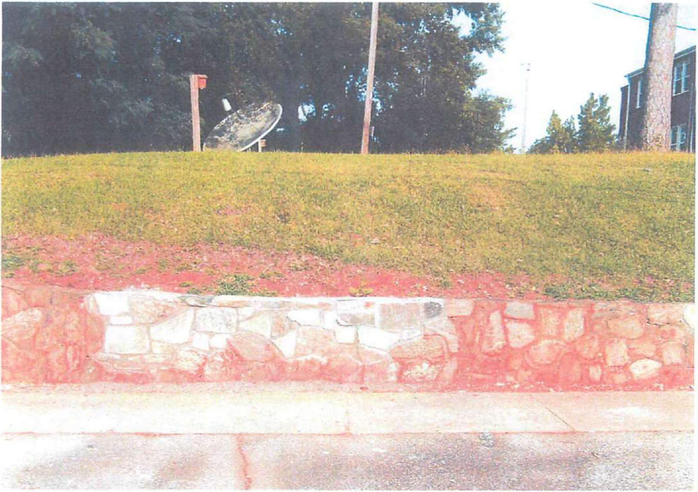
Stone wall on South Church Street - AFTER
